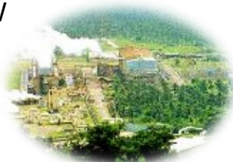
Tiwi Complex 290 MW
